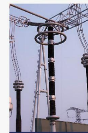
1000kV UHV AC Station Arrester MOV Model: DI28
