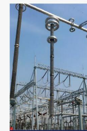
±800kV UHV DC Converter Station Arrester MOV Model: DI15
