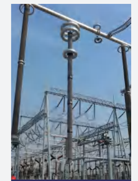
±800kV UHV DC Converter Station Arrester MOV Model: D115
